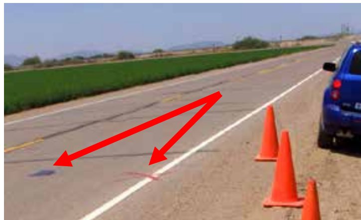
Figure 7. Deployed Hi-Star at a Two-Lane Site
